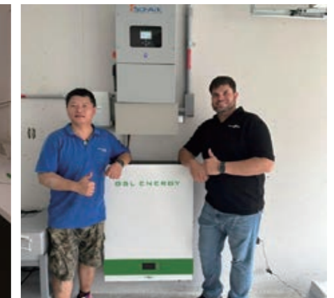
-Puerto Rico 14.34kWh Hybrid Solar Storage System
